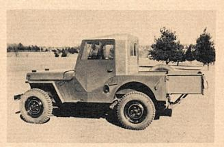
RANCHERS, STOCKMEN, AND FARMERS ARE FINDING THE PORTER & REED ALL-METAL HALF BODY INVALUABLE IN THEIR TYPE OF WORK... THE HALF BODY ALLOWS FULL USAGE OF ALL JEEP ATTACHMENTS AS WELL AS THE EXTENSION BED AS SHOWN IN THE PICTURE... THE BACK PANEL CAN BE EASILY REMOVED TO ALLOW WORKING OF LEVERS AND ROPES. SIDE DOORS CAN BE TAKEN OFF IN A FEW MINUTES FOR COOLER DRIVING AND WORKING IN THE SUMMER TIME.
