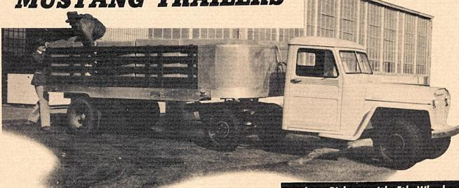
The Mustang Trailer meets the long recognized need for a light, conventional type trailer that can be handled by a JEEP. Interchangeable sides and nose make it adaptable for hauling any conventional load . . . grain, livestock, and general produce.
