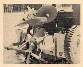
Here the Fire Fighter Plow is shown in transit position with most of the weight off the lift and supported by the 'Jeep.'
